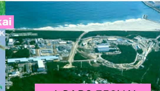
J-PARC 750kW (under construction)
