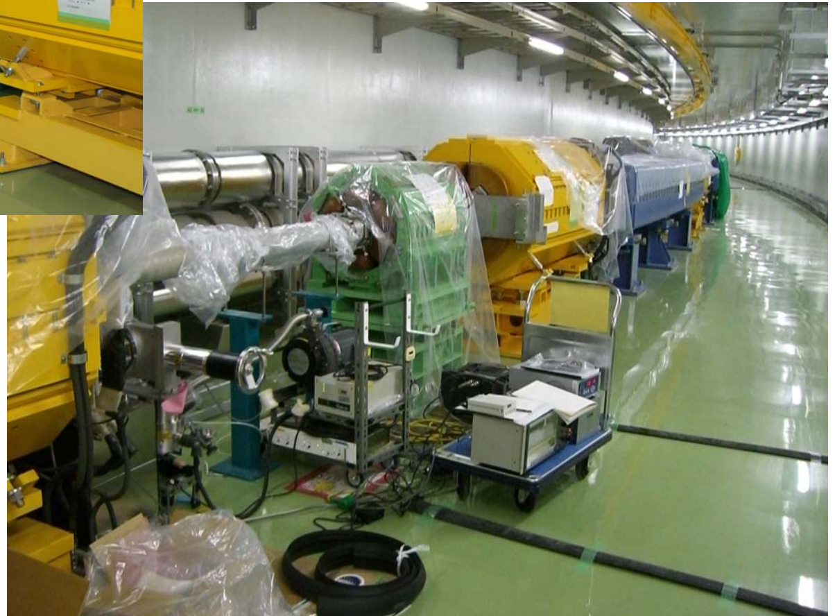
Vacuum evacuation test at Arc-B
