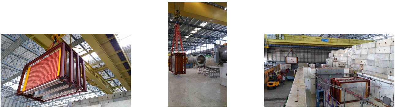
Figure 14: Left: Lifting Baby MIND chassis 1 to the beamline at the PS. Middle: Chassis 1 approaching the Proton Synchrotron (PS) experimental hall. Right: Chassis 2 approaching the PS hall.
